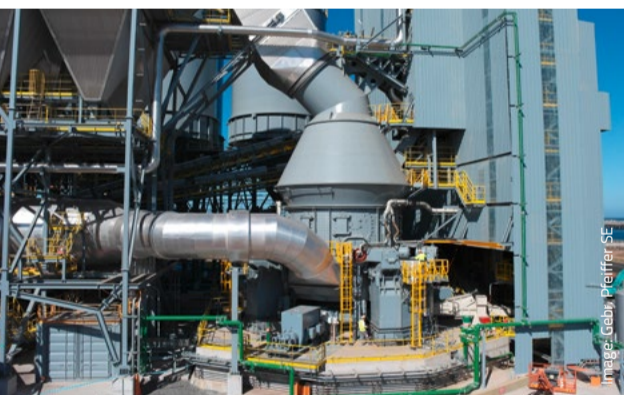
> Australia's largest cement mill
